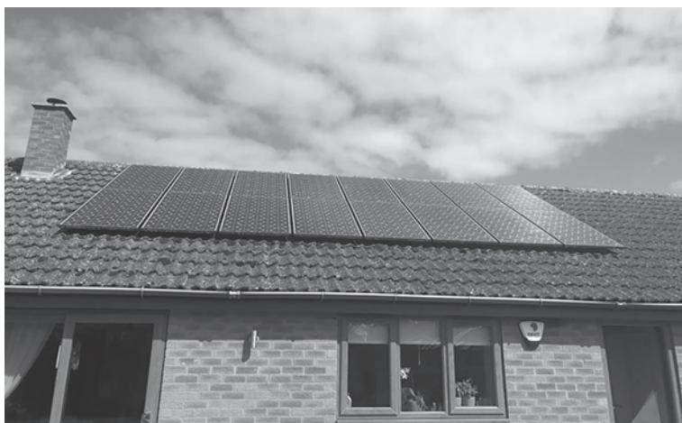
Solar panel efficiency is the percentage of solar energy the solar panel converts to electricity on a sunny day with temperatures of 25 °C.
