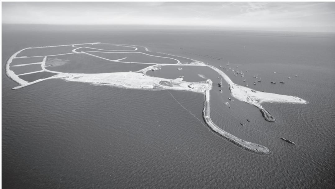
(a) Clay, sand and silt from the bottom of the lake was used to make these islands.
