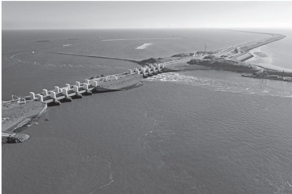
Afsluitdijk dam was built in 1932. The dam is a sea defence that encloses a salt-water inlet of the North Sea. The dam is 7.25m above sea level, 90m wide and 32km long. It protects the land from flooding.
